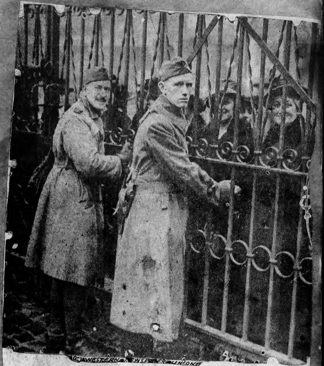
Crowds at the gate of the pier at Hoboken, eager to embrace their loved ones in the 57th as they returned from the battlefields aboard the Huntington.
