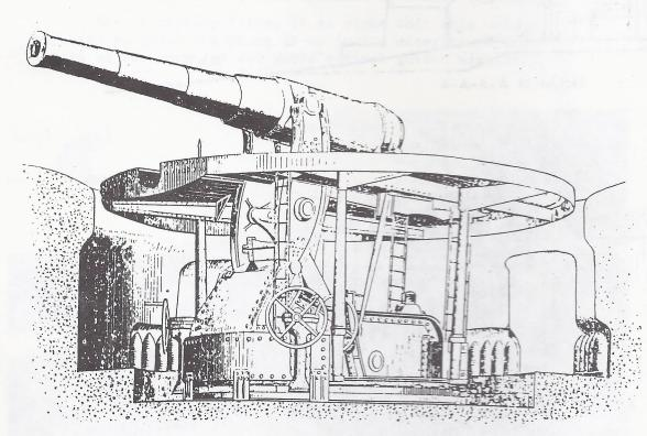
ABOVE: A disappearing coast gun concealed within a concreted pit and covered with an iron shield. The gun is down, for loading.
